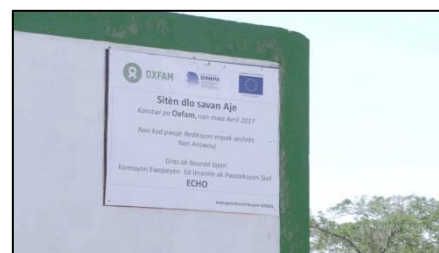
Water storage tank in Anse Rouge (North-West). Photo: ECHO
