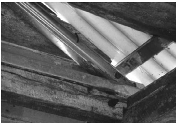
Photos 20. Detailed connection of metal structures of the new roofs on pre-existing structures applying various on-site solutions
