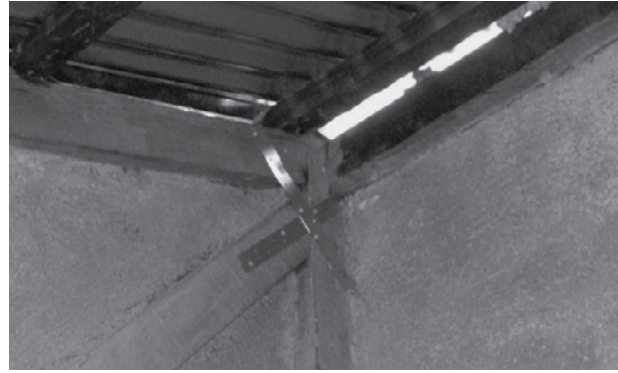
Photo 16. Strapping loop-type connection: the ends can be crossed and fastened at each end with at least 2 nails
