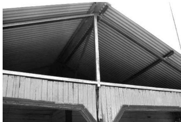
Photos 8 to 10. Detailed assembly and installation of new metal frame and roofing elements on wooden elements of the houses under rehabilitation
