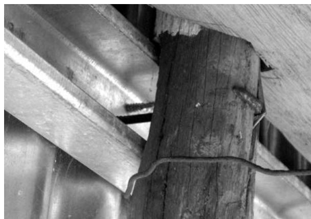
Photos 20. Detailed connection of metal structures of the new roofs on pre-existing structures applying various on-site solutions
