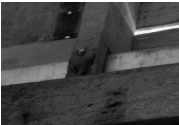
Photos 17 to 19. Connection of metal frameworks or falseworks with wooden beams using screws
