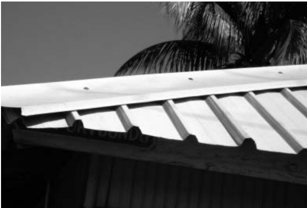
Photos 4 and 5: View of cross-gabled roofs with fretted metal tiles and supplementary pieces on ridges and junctions of sloping planes
