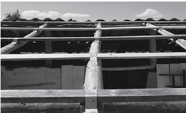
Photos 13 to 15. Connection of beams and purlins: 2 nails minimum at each end and on the beam
