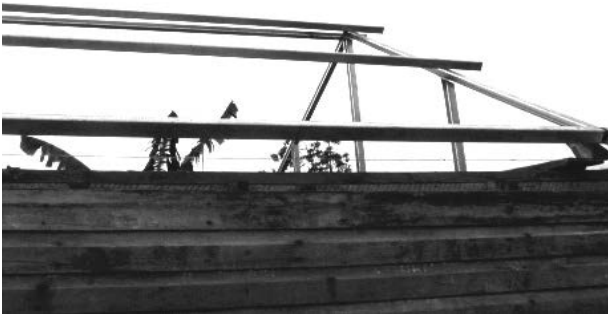
Photo 7. Framework or falsework with profile joists or purlins ready to be mounted on the wooden structure of a house under rehabilitation
