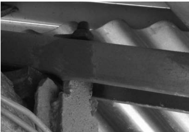
Photos 11 to 16. Detailed connection of metal frameworks or falseworks of the new roof on pre-existing wooden beams, using steel plates and threaded screws
