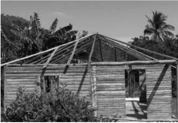
Photo 6. Levelling and preparation of bearing structure on one of the houses to be rehabilitated
