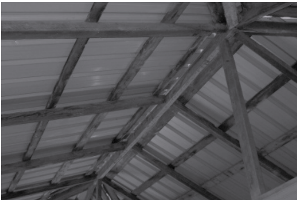
Photos 8, 9 and 10: Re-use of original structural elements on masonry (brick and block) houses
