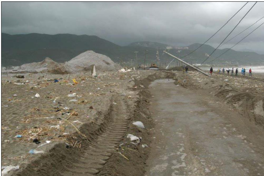
Plate 6.1: Sediments deposited along the Palisades roadway after Hurricane Ivan (2004). Source: NWA 2012.
