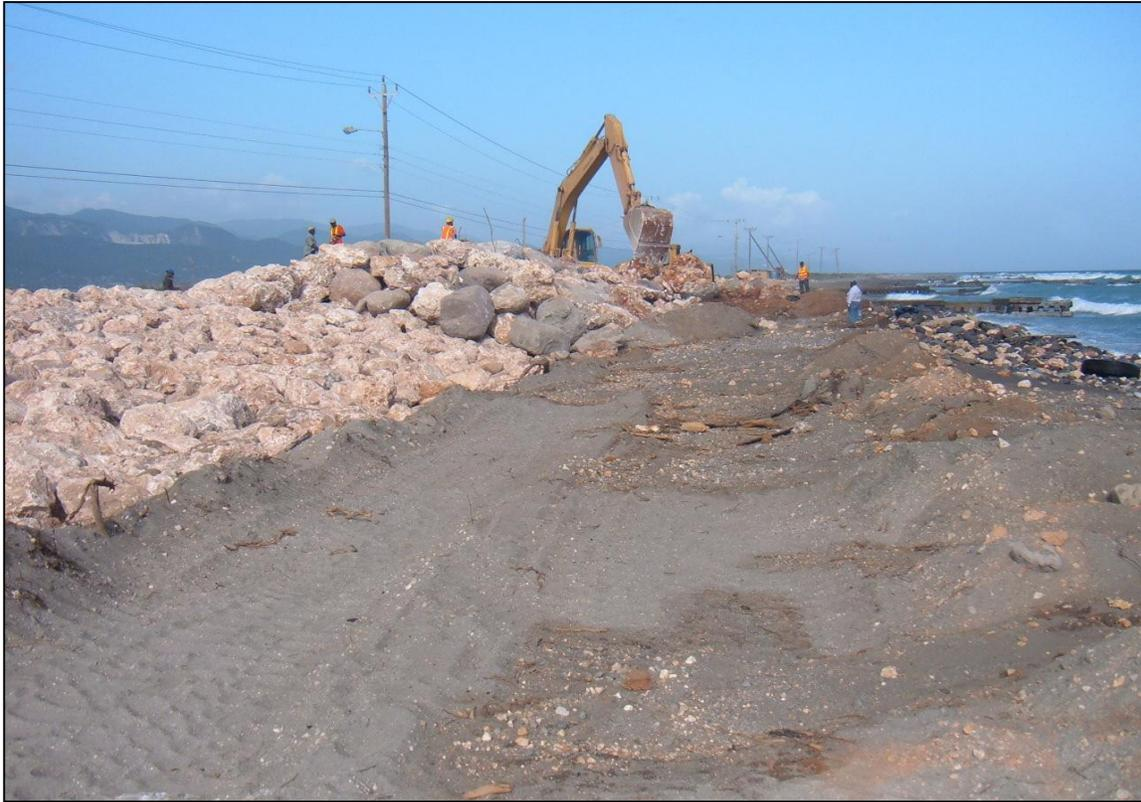
Plate 6.2: Protection of the Palisadoes roadway. Source: NWA 2012.
