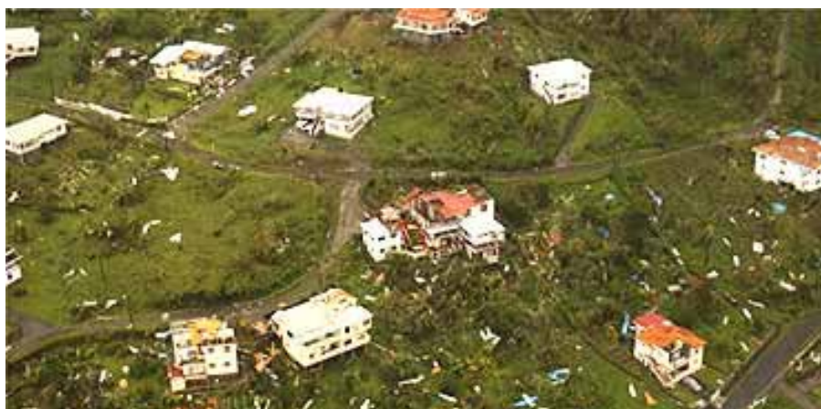
Figure 10. Buildings in Grenada Damaged by hurricane Ivan
