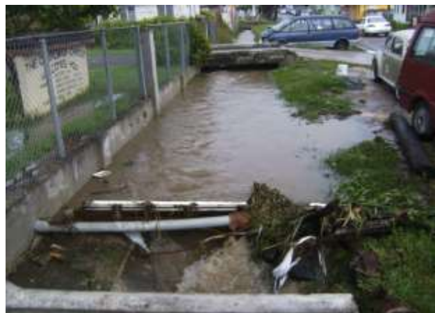
Fig: 42 Littering/illegal dumping blocking drains Source: NODS
