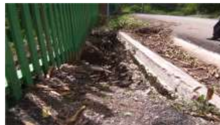
Fig: 35 Potential road undermine and collapse: Source NODS
