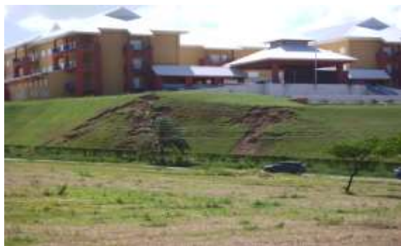
Fig: 47 Slope instability after heavy rains 2008
