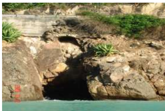
Fig: 46 Erosion undermining road Crabbe Hill, Source: NODS
