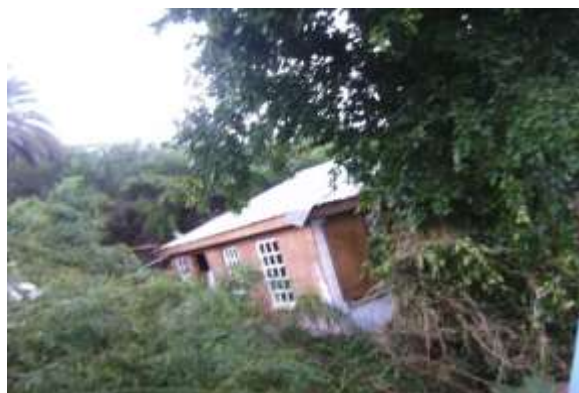
Fig: 44 House relocated by stream flood waters, Buckley Line Source: NODS
