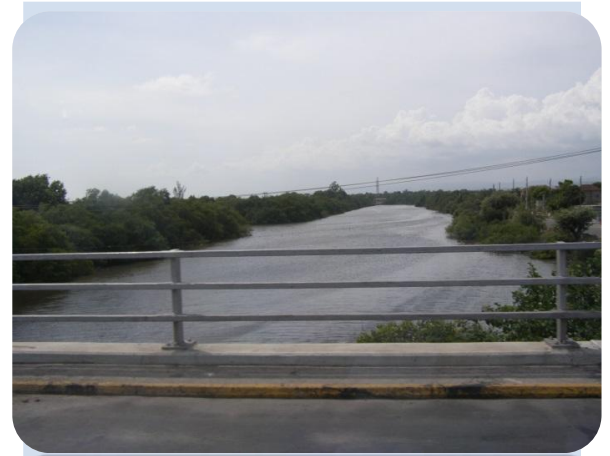
Large Canal that contribute to flooding
